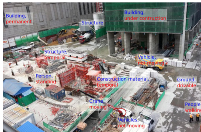
Fig. 5. Semantic understanding allows humans to predict changes in the environment at different time scales. For instance, in the construction site shown in the figure, humans account for the motion of the crane and expect the crane-truck not to move in the immediate future, while at the same time we can predict the semblance of the site which will allow us to localize even after the construction finishes. This is possible because we reason on the functional properties and interrelationships of the entities in the environment. Enhancing our robots with similar capabilities is an open problem for semantic SLAM.
